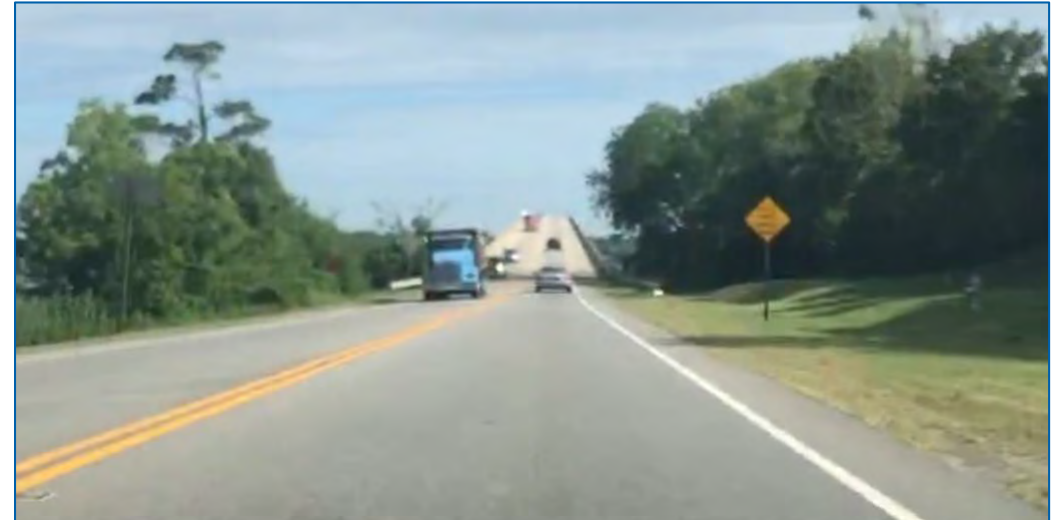
US 17 Northbound Shoulders on Godwin Jr Bridge Approach
