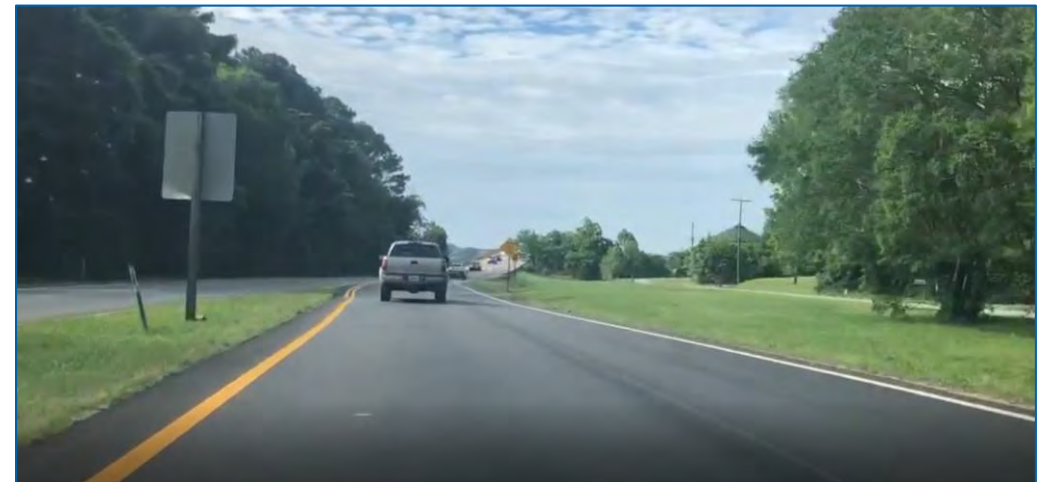
US 17 Southbound Shoulders on Godwin Jr Bridge Approach
