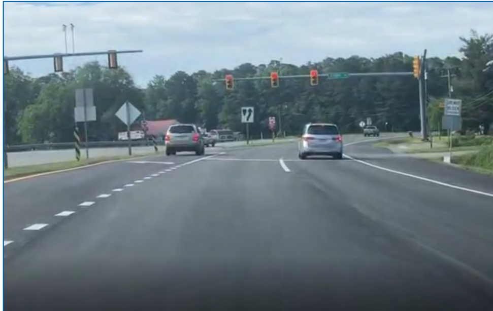
High-Vis Backplates / Newer Pavement (Overlay) / Pavement Markings
