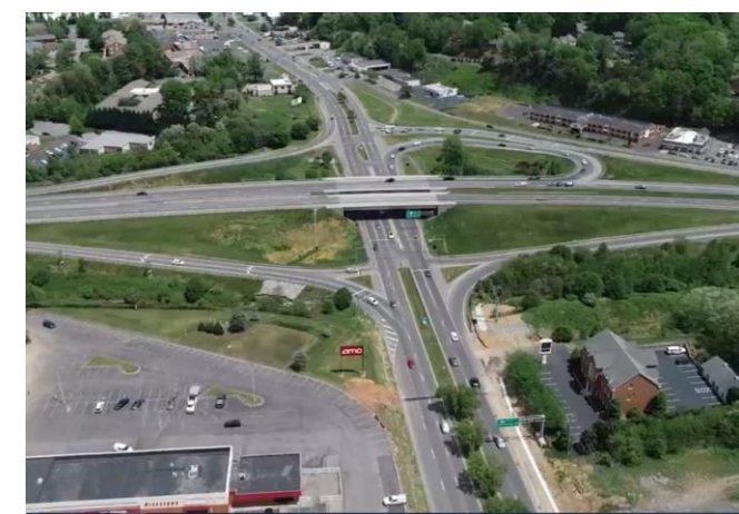
Route 419 and Route 220 interchange
